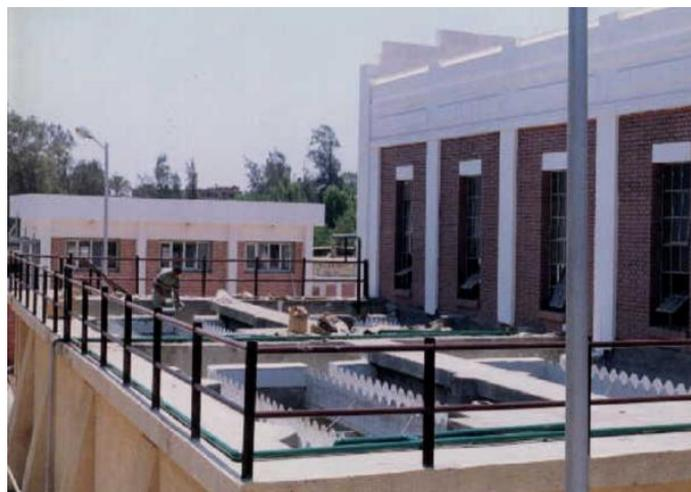
**Photo 4** The upgraded rectangular sedimentation tank.
