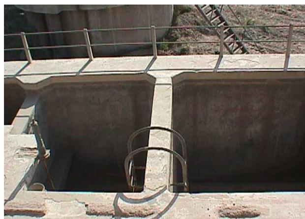
**Photo 2** Rectangular sedimentation tanks (no. 2 &3)
