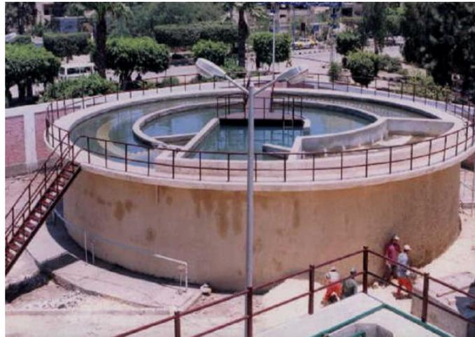
**Photo 3** The upgraded circular sedimentation tank.
