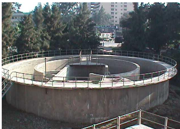
Photo 1 The circular sedimentation tank (no.1)
