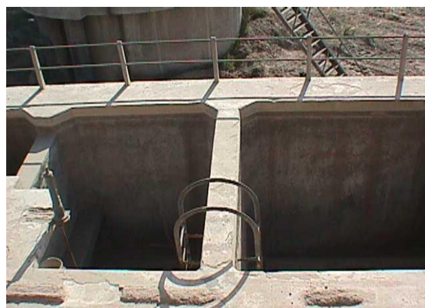
Photo 2 Rectangular sedimentation tanks (no. 2 &3)
