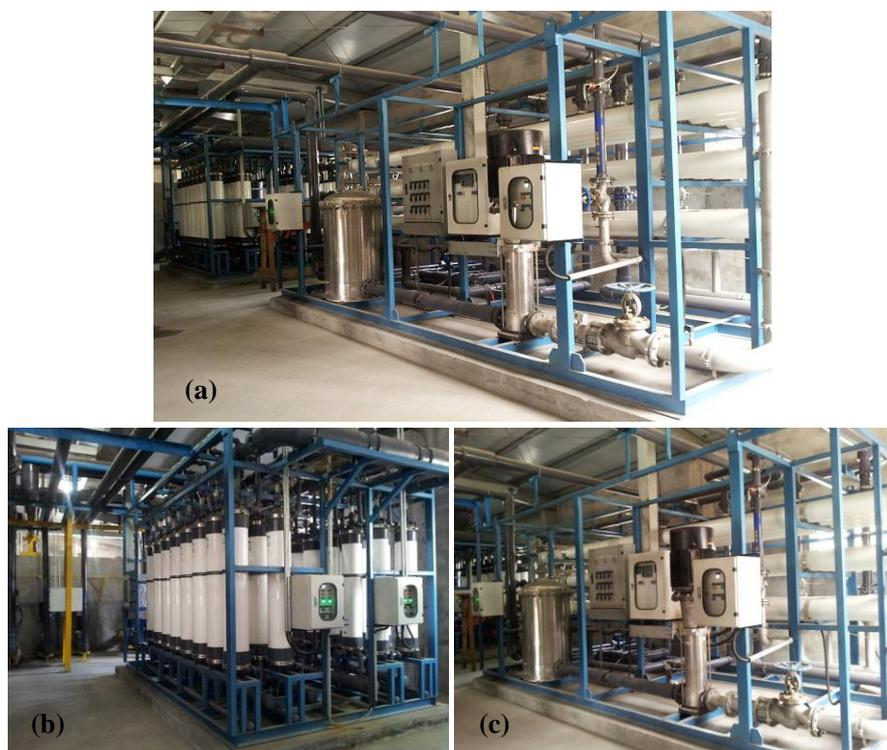
**Figure 2** The photographs of the full-scale electroplating wastewater treatment plant: (a) a full view of the integrated UF/RO system (b) UF installation, (c) RO installation
