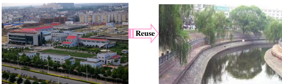
Figure 1 The on-site picture of the full-scale municipal plant
